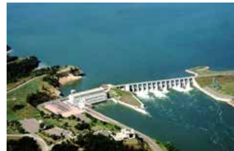
Gavins Point Dam 4
